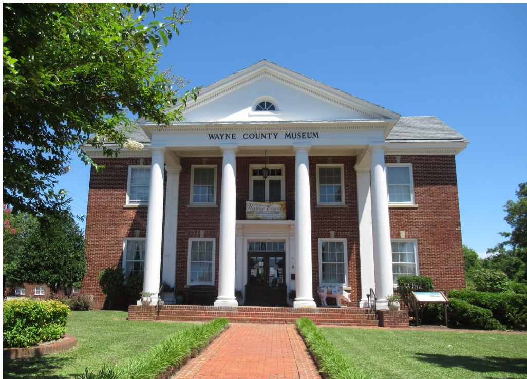
Façade, View to East
