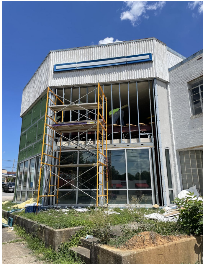
Oblique front view of showroom to east
