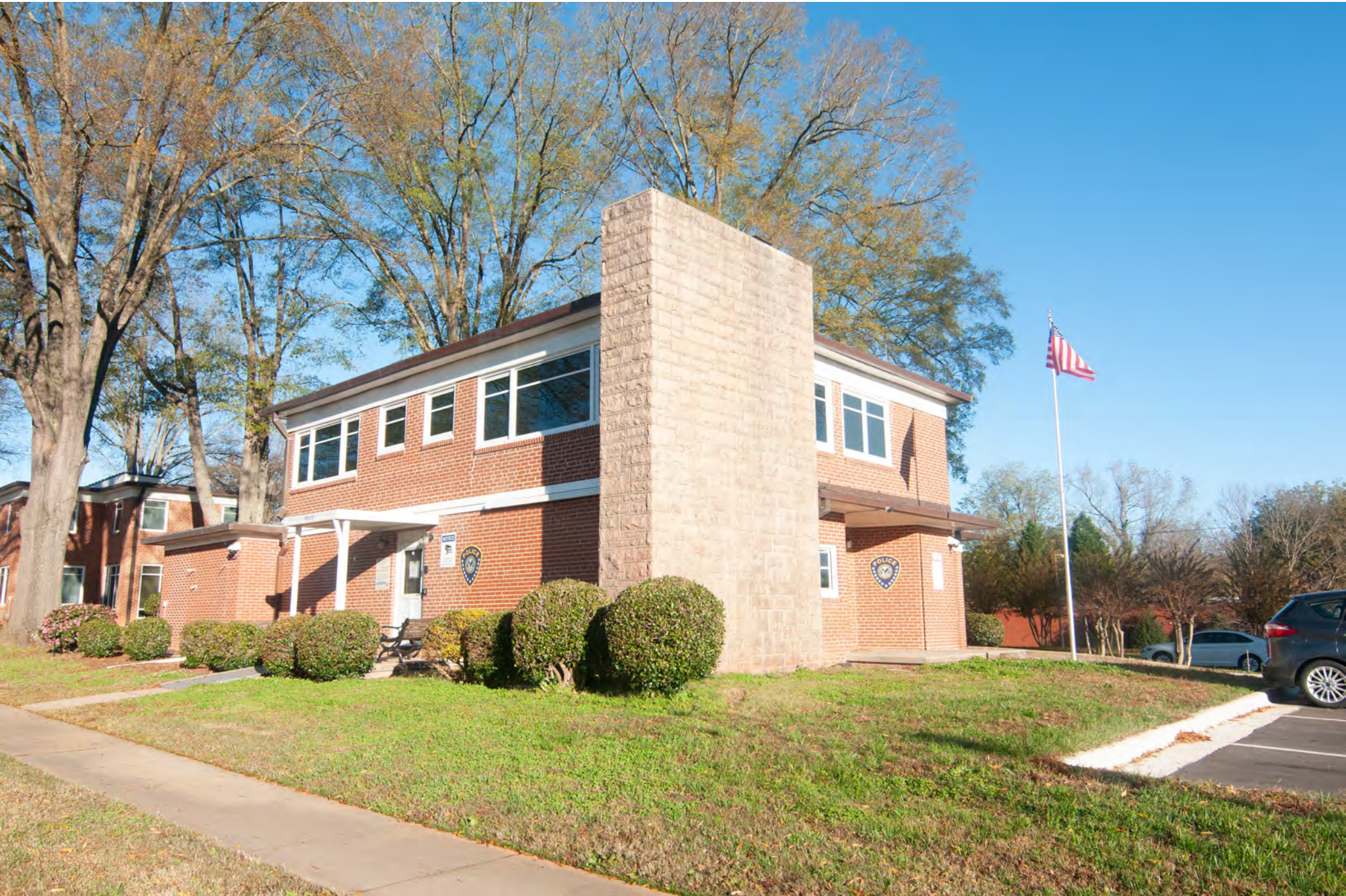
Photo 18 of 55.Salisbury VA Hospital Historic District, Salisbury, Rowan County, North Carolina. March 2021.
