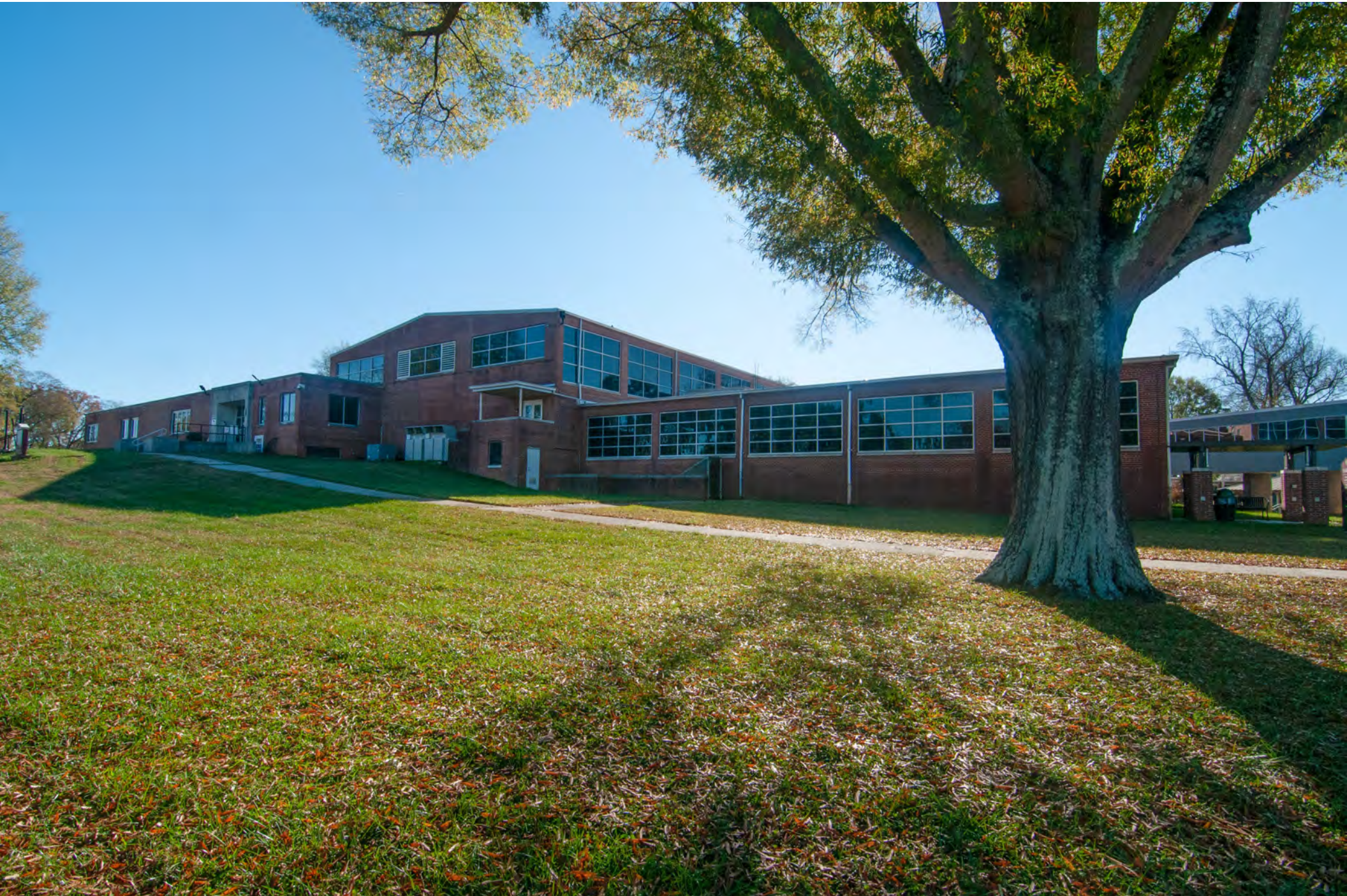
Photo 9 of 55.Salisbury VA Hospital Historic District, Salisbury, Rowan County, North Carolina. March 2021.
