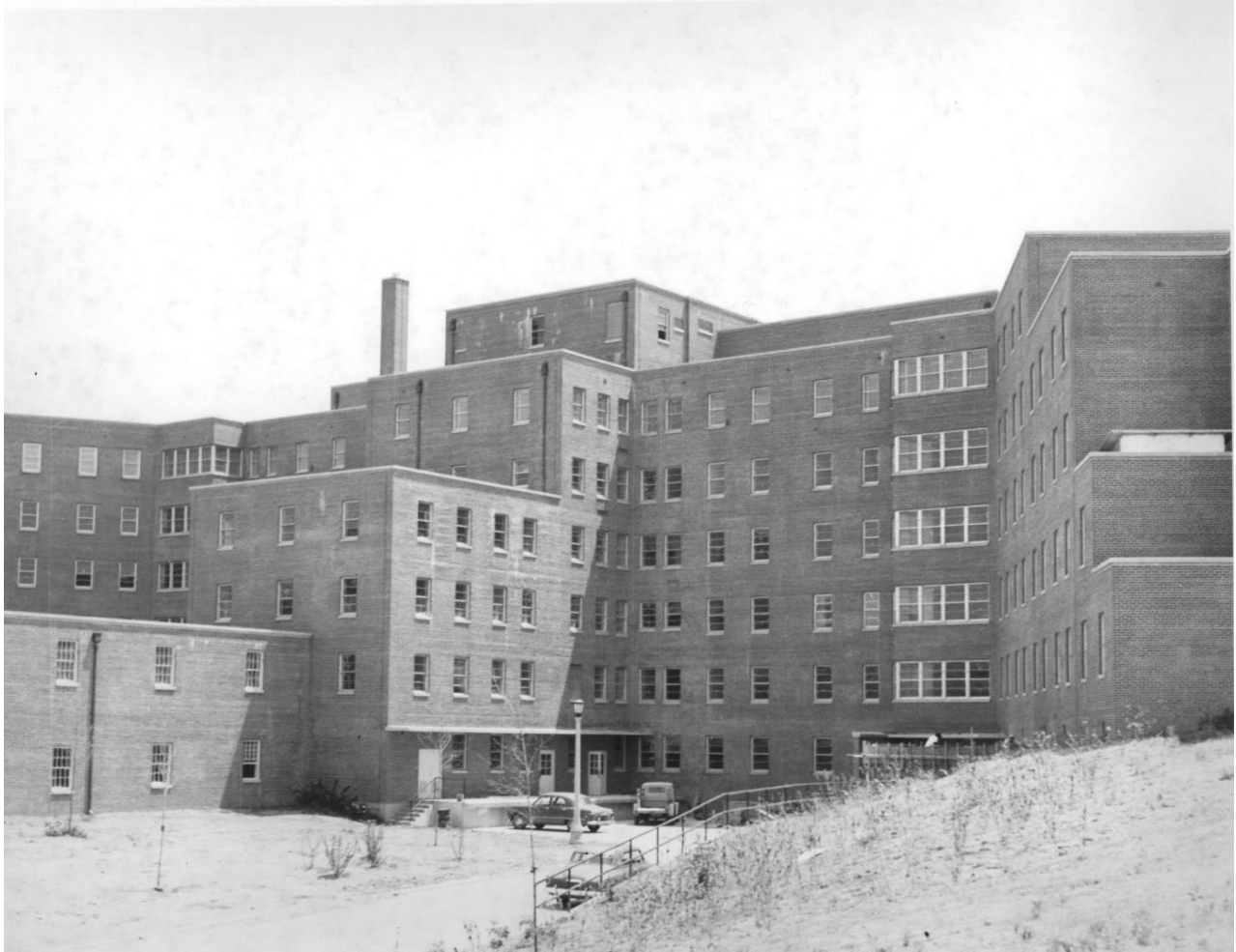
Figure 1: Rear elevation of Building #2, June 1953. Collections of Federal Preservation Office, U.S. Department of Veterans Affairs, Washington, D.C.
