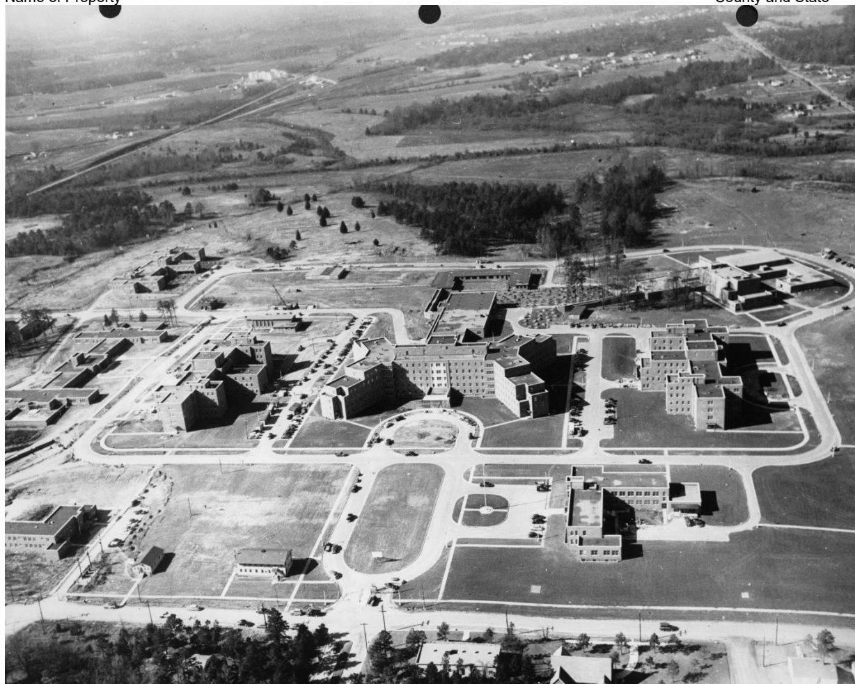
Figure 3: View of Salisbury VA Hospital, ca. 1953. Collections of Federal Preservation Office, U.S. Department of Veterans Affairs, Washington, D.C.
