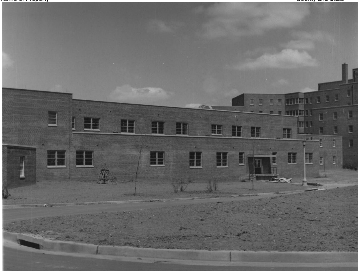
Figure 2: View of Building #5, April 1953. Collections of Federal Preservation Office, U.S. Department of Veterans Affairs, Washington, D.C.
