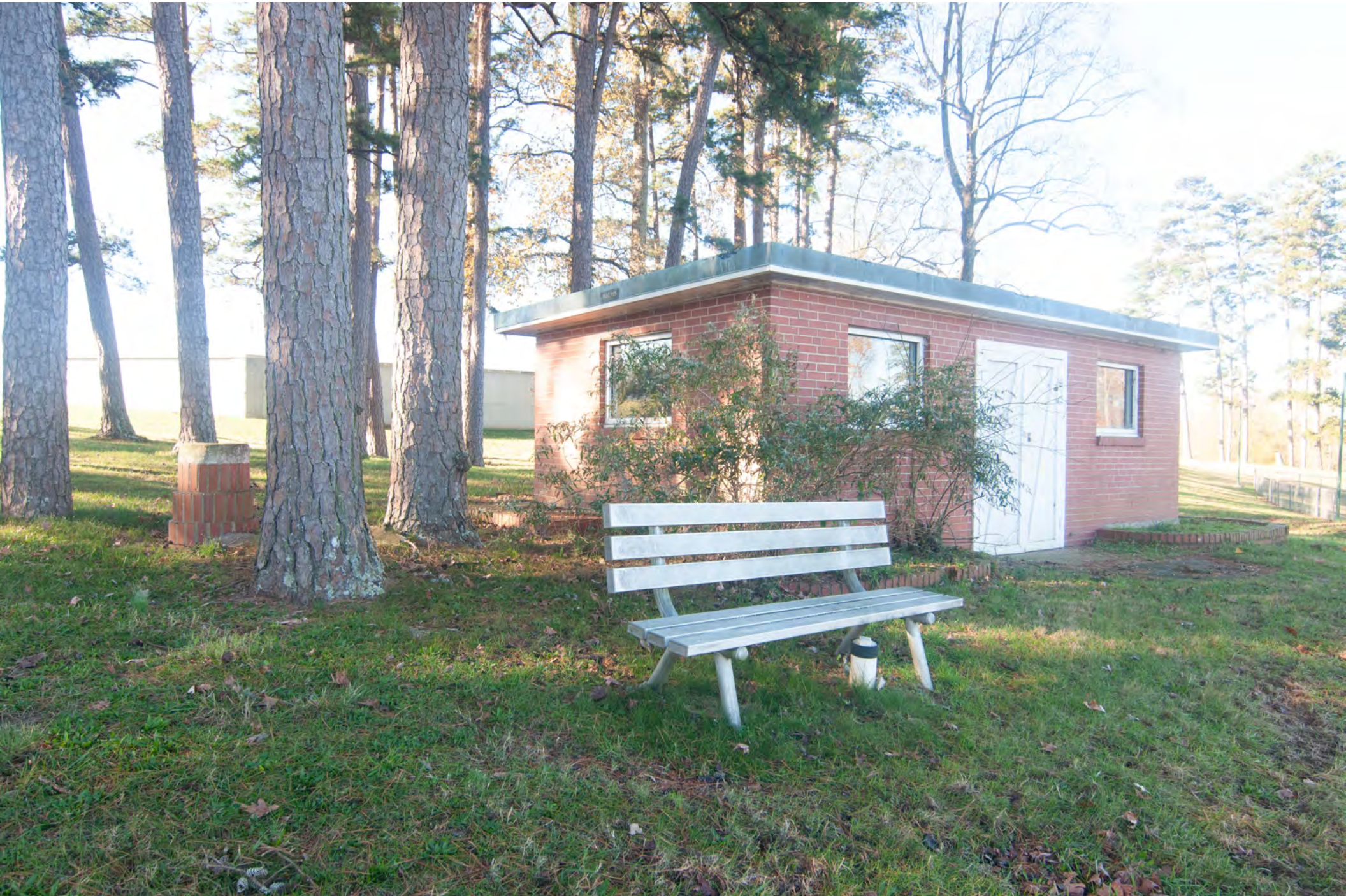
Photo 39 of 55.Salisbury VA Hospital Historic District, Salisbury, Rowan County, North Carolina. March 2021.
