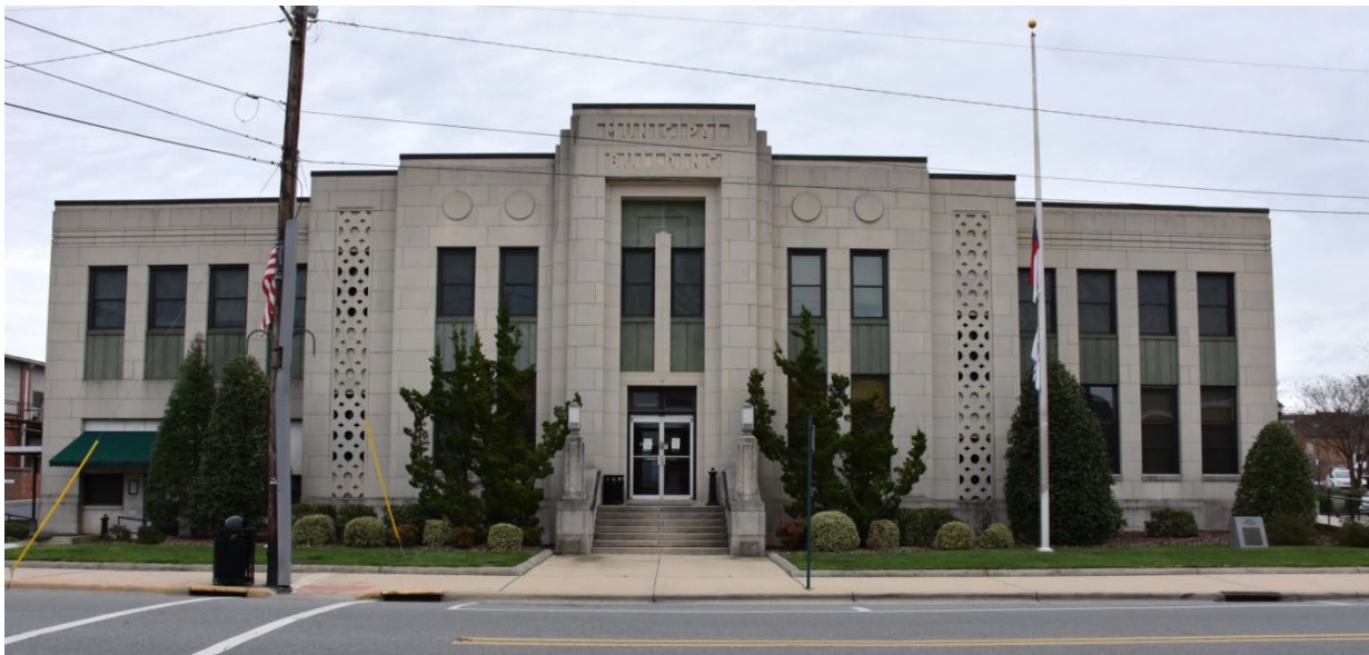
6. Asheboro Municipal Building, 1939, circa 1957, 146 N. Church Street (below)
