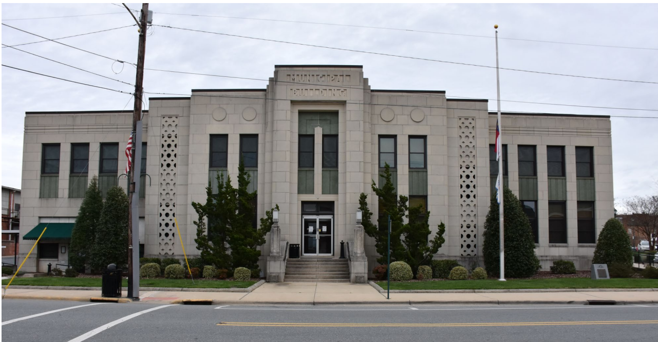
Asheboro Municipal Building, 1939, circa 1957, 146 N. Church Street
