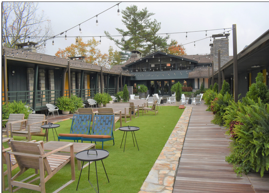
2. Skyline Lodge, Main Lodge Building and Courtyard, North Elevation, facing south.
