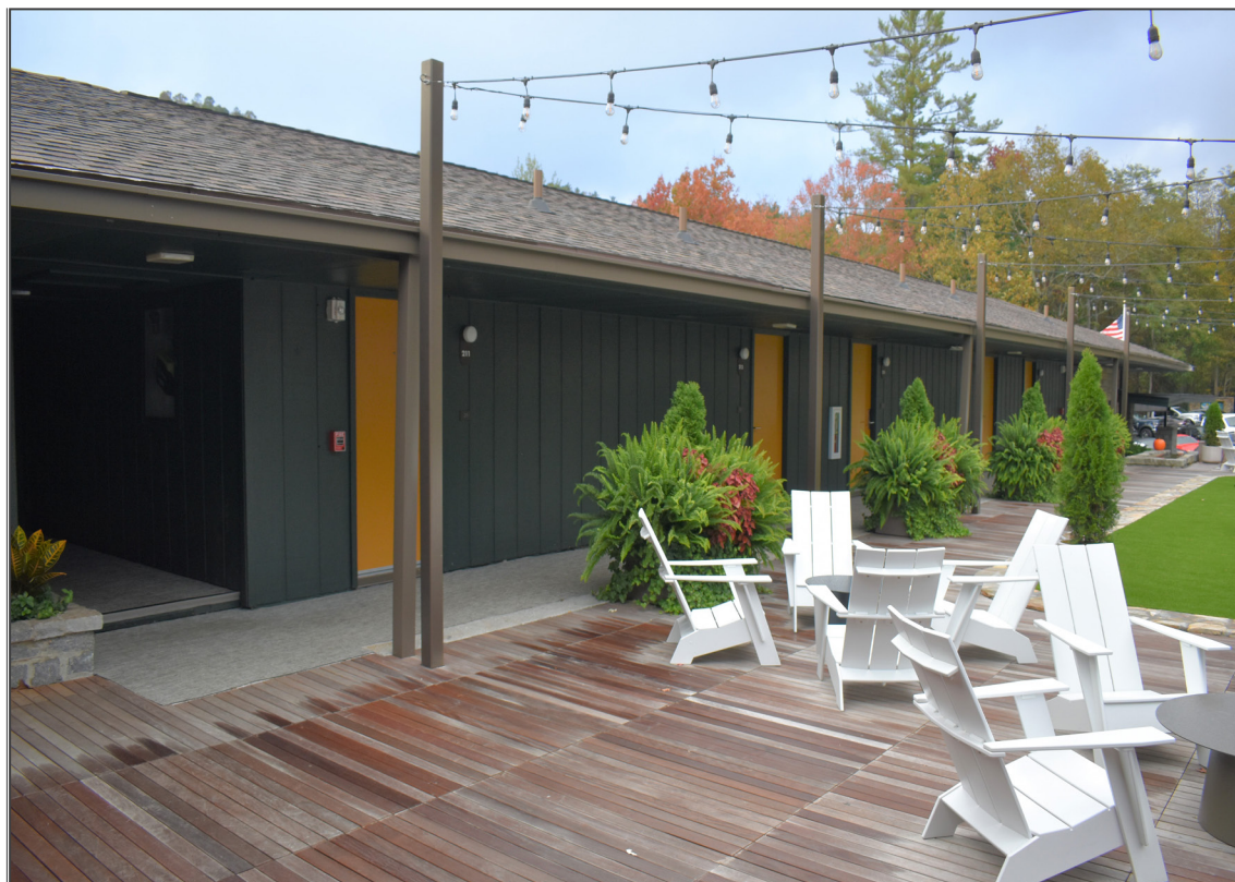
10. Skyline Lodge, Garage Guest and Service Wing, East Elevation, facing northwest.
