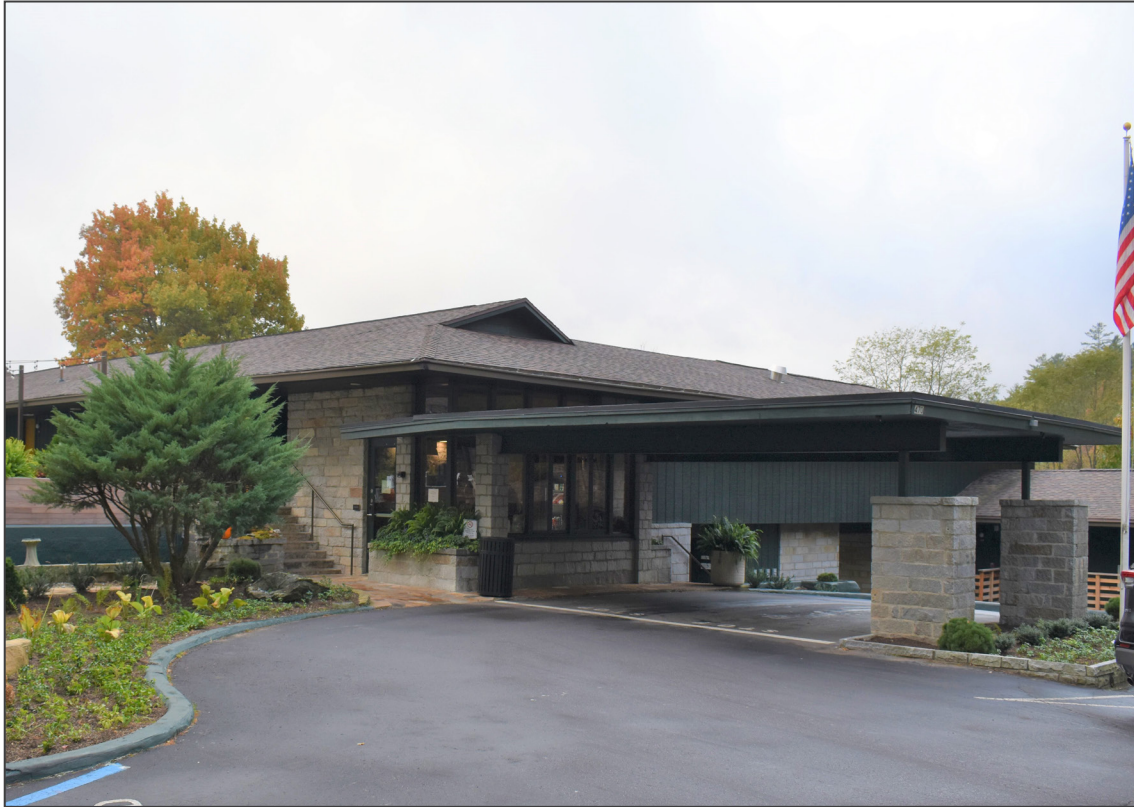
13. Skyline Lodge, Reception and Porte Cohere (1965), facing southwest.
