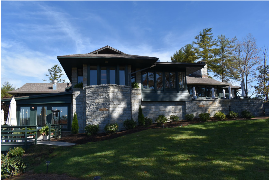
South Elevation, facing north
