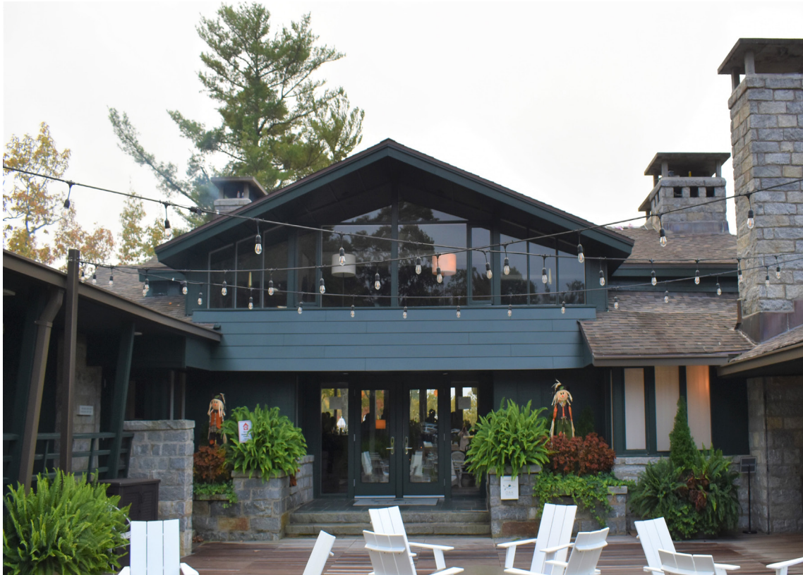
3. Skyline Lodge, Main Lodge, North Entrance and 1965 Gable Addition, facing south.
