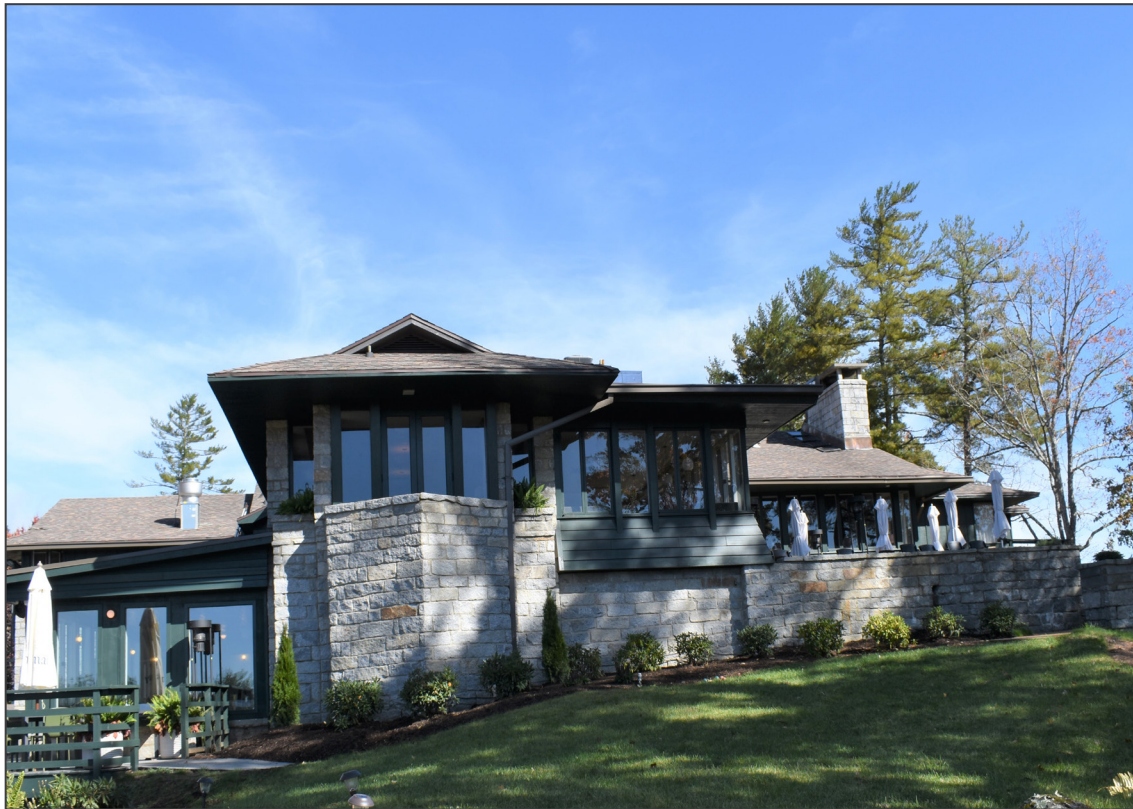
1. Skyline Lodge, South Elevation , facing north.
