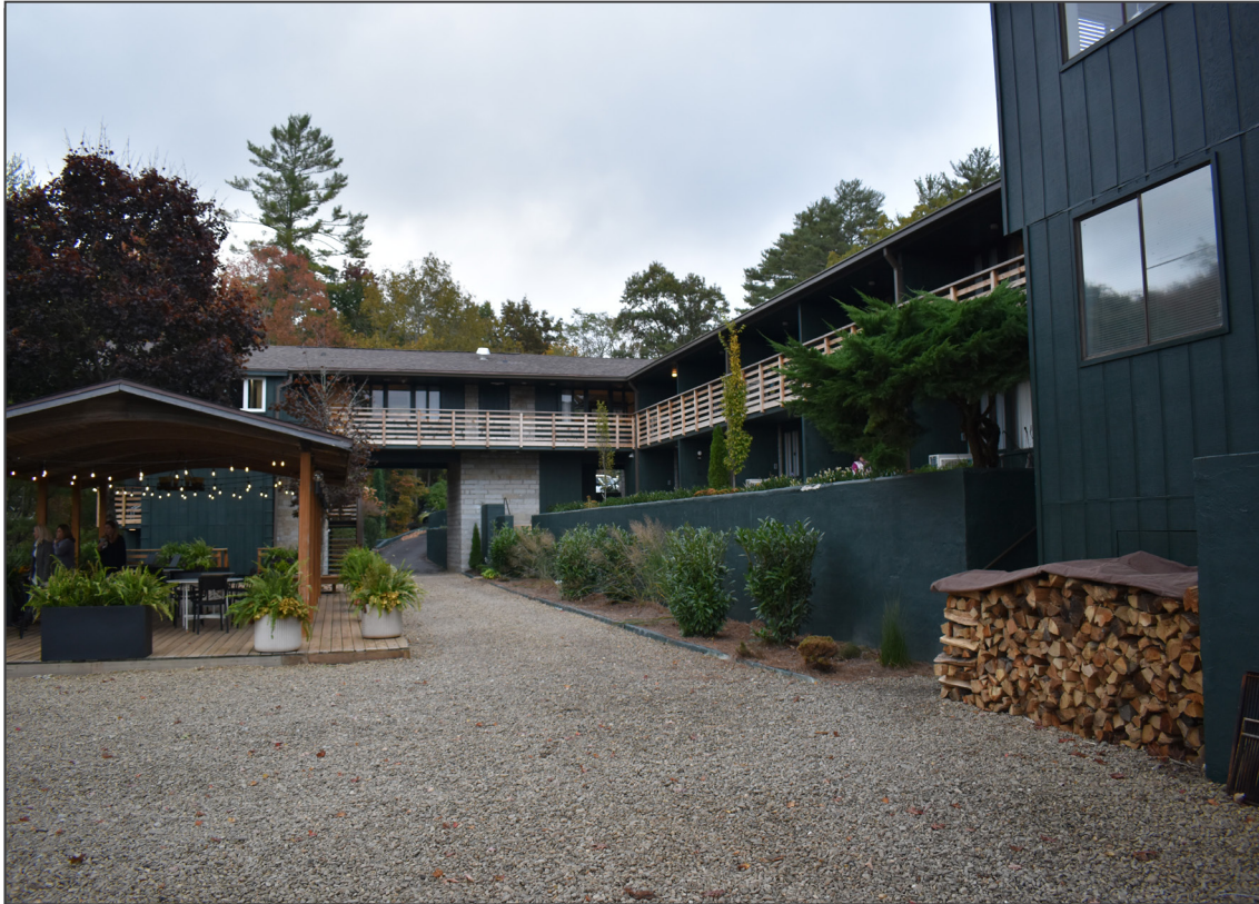
11. Skyline Lodge, Garage Guest and Service Wing, West Elevation, facing northeast.
