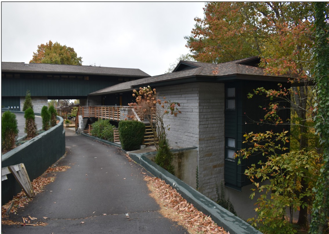
14. Skyline Lodge, Garage Guest and Service Wing (L) and Opsahl Guest Wing (R), East Elevation, facing southwest.
