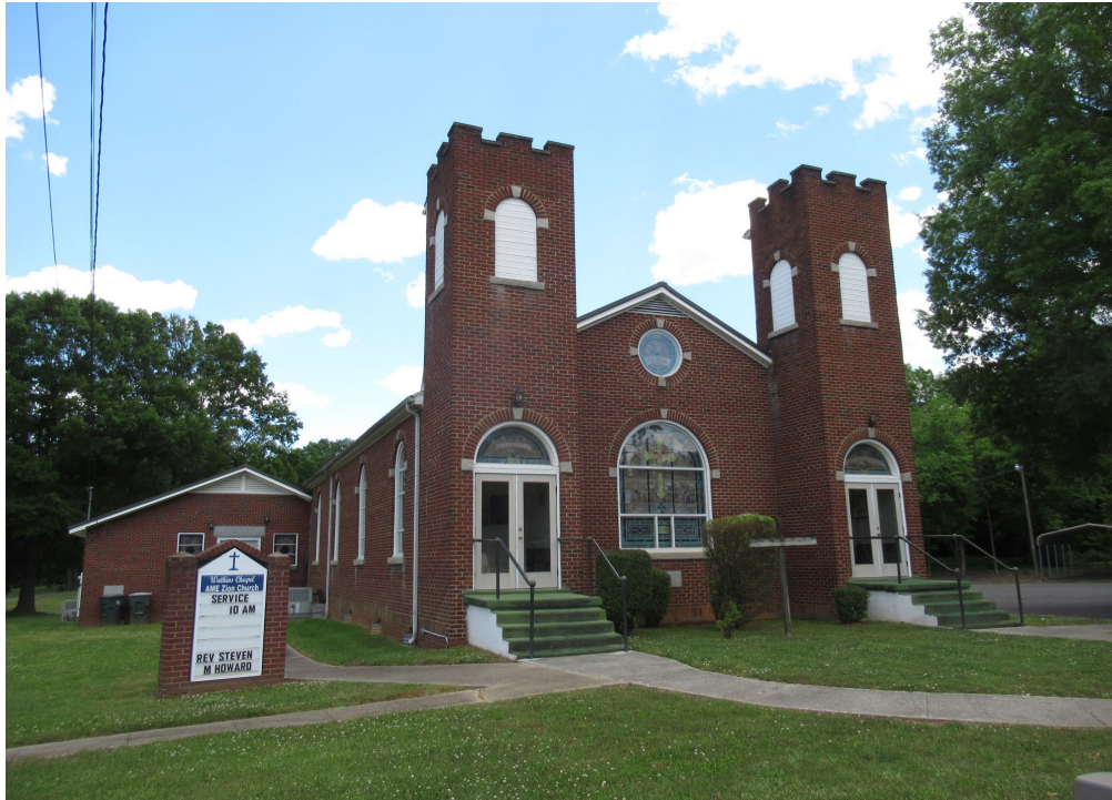
Church, exterior, facade, view to southeast
