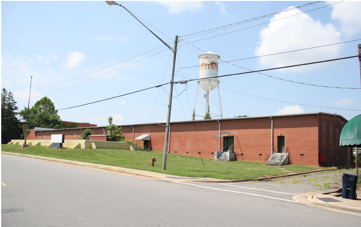
1892 Stanley Creek Cotton Mill/Lola Mill No. 1, East Façade, Camera Facing Southwest
