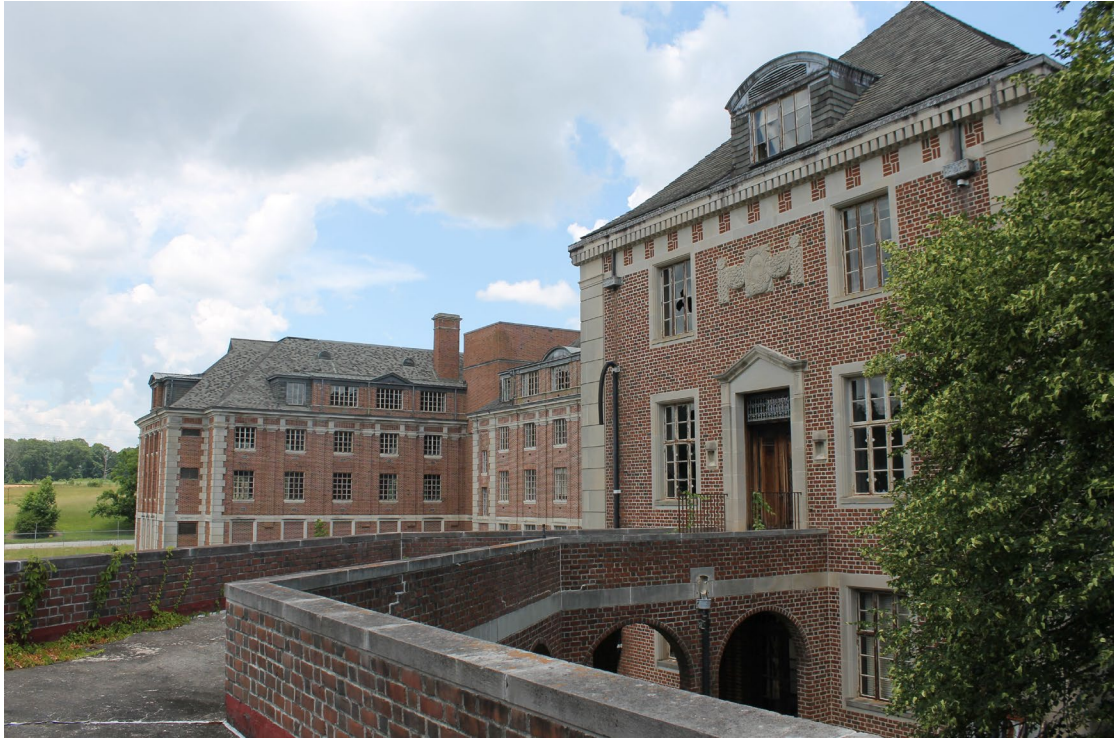
Fackler Building, west end with the Annex and North Buildings in distance
