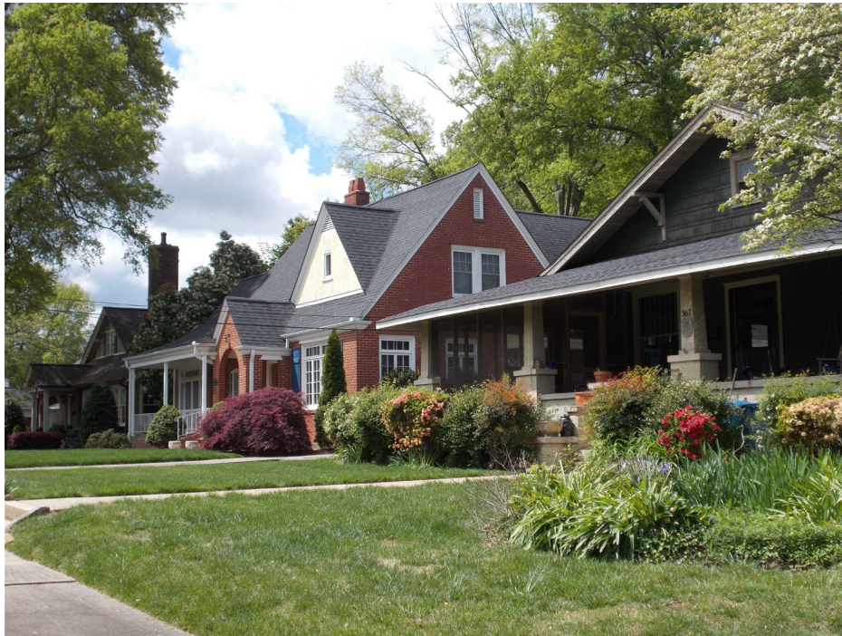
300 block of 7th Street NW, west side. View facing southwest
