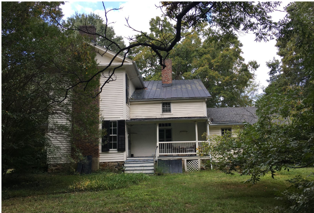
East facade, camera facing west
