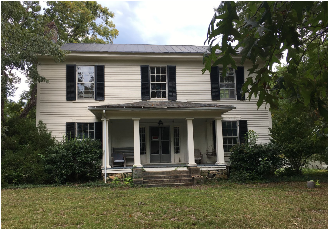
South facade, camera facing north
