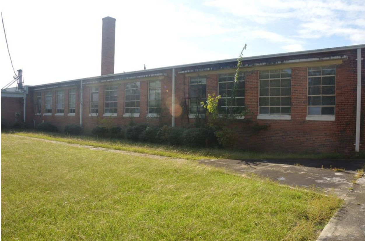
Front of building/ East View
