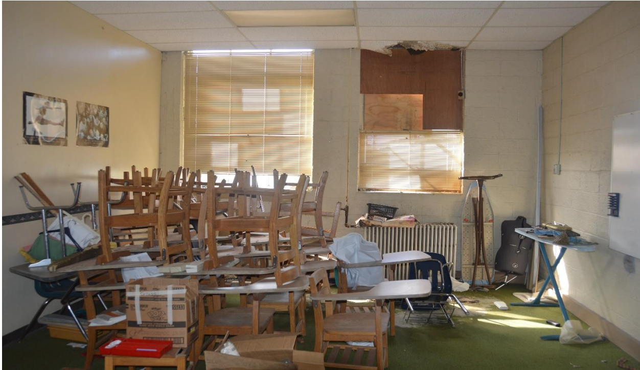
Westside Classroom on east of corridor
