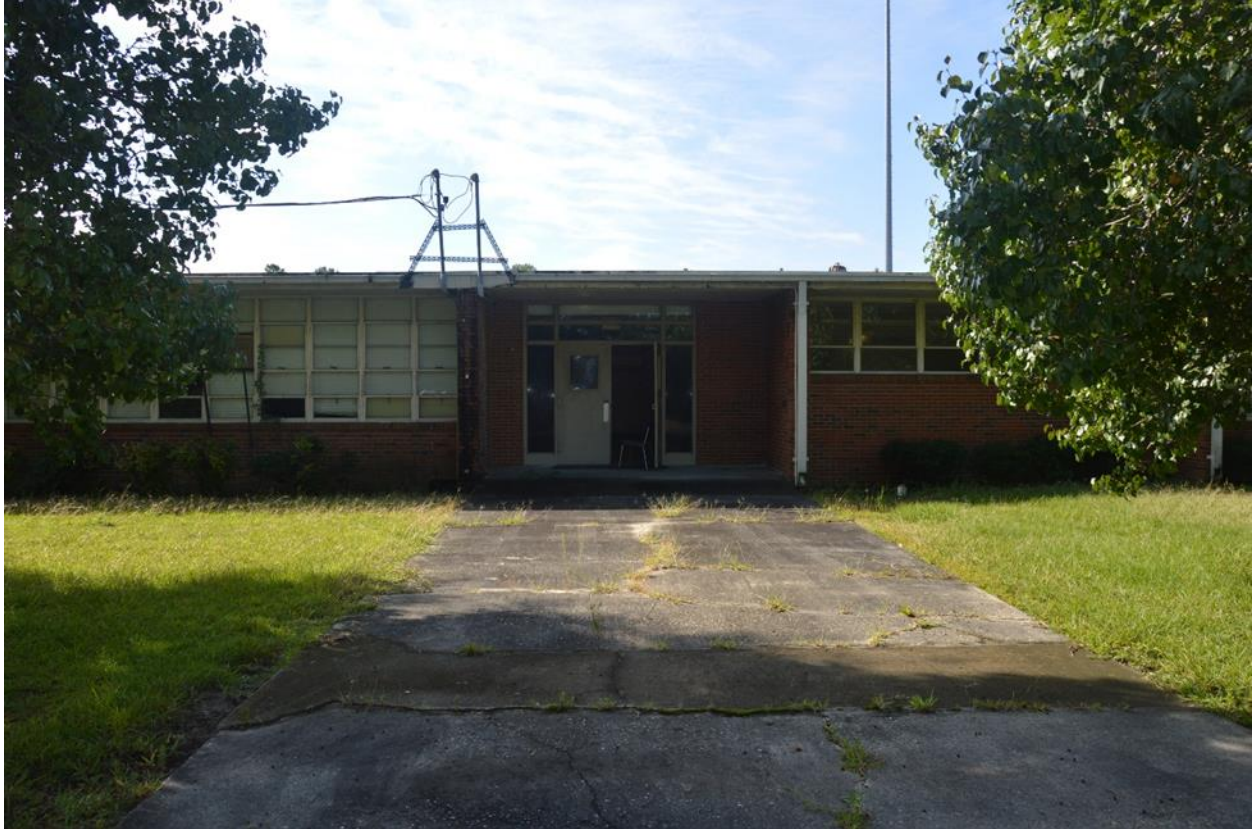
Westside Entrance/Exit Foyer Northwest
