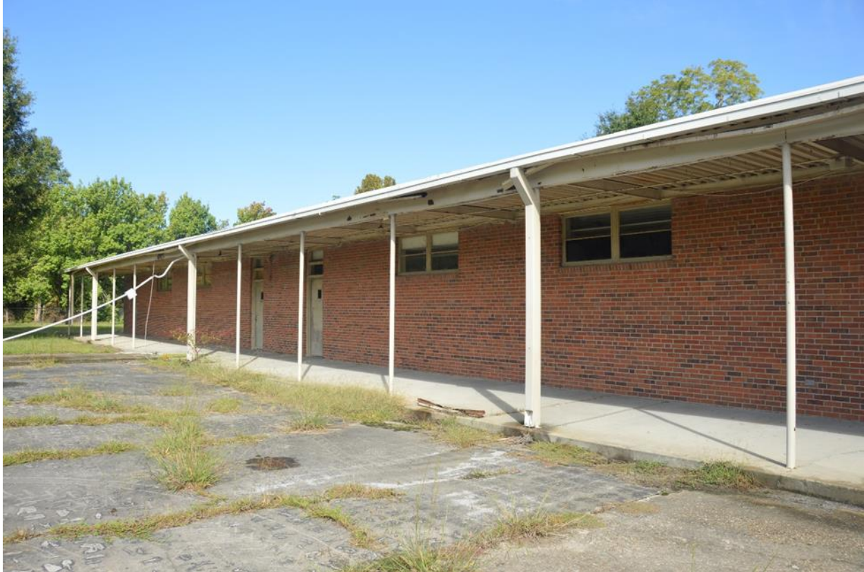
Westside Rear of School Classroom Building
