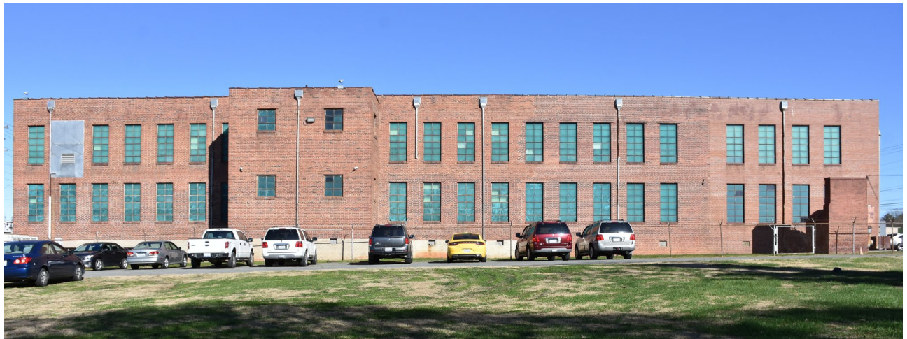
1946 and 1951 additions, west elevation with incinerator at right
