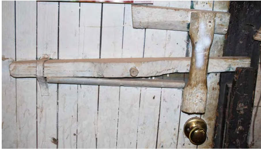
BK0364, Store, 1910s, 6127 US 64, Morganton vicinity Interior latch on double-thickness front door (diagonal boards on the exterior, vertical boards on the interior)
