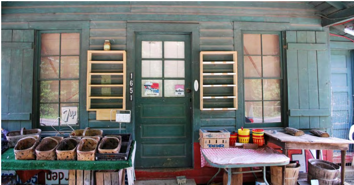
BK0380, Mull Store, 1931, 1651 N. Green Street, Morganton Board-and-batten shutters provide additional security for façade windows when closed
