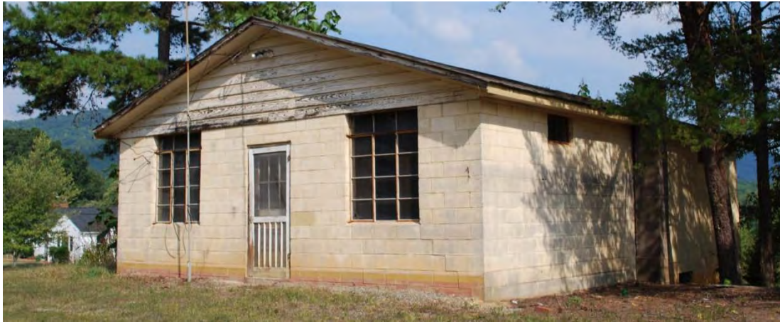
RF0463, Freeman Store, ca. 1951, 3490 Bostic-Sunshine Highway, Bostic vicinity
