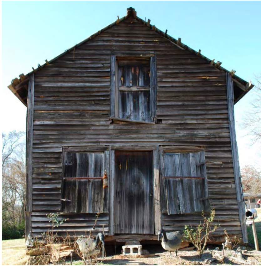
BK0263, Tilley Store, 2599 Smokey Creek Road, Drexel vicinity Board-and-batten shutters cover the six-over-six sash windows (above) Metal interior bars provide additional security (below)
