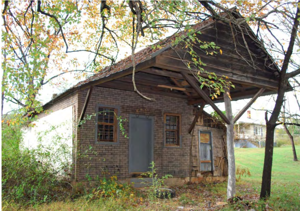
MC0200, Store, 1930s, Montford Cove Road, Montford Cove vicinity
