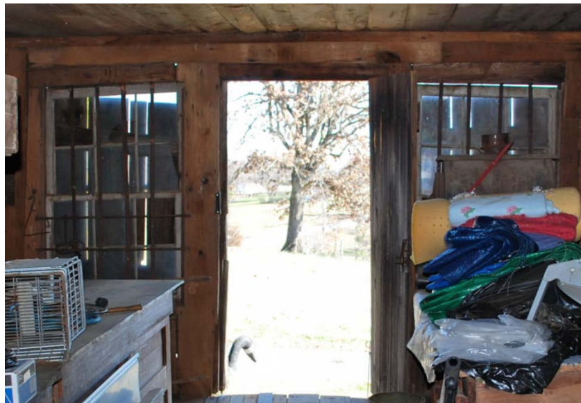
BK0263, Tilley Store, 2599 Smokey Creek Road, Drexel vicinity Board-and-batten shutters cover the six-over-six sash windows (above) Metal interior bars provide additional security (below)
