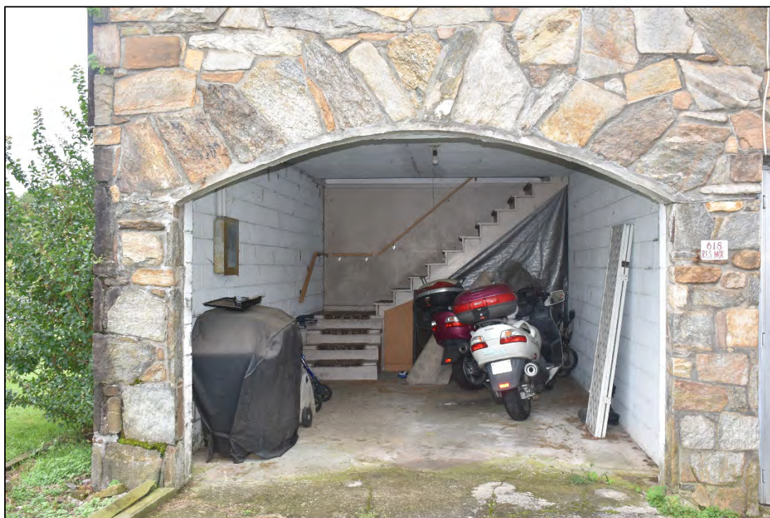
Figure 2.22. Meadow's Store and Apartments (BN6343), apartment garage detail, facing south.
