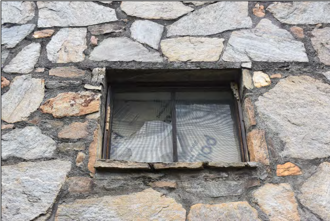
Figure 2.8. Meadow's Store and Apartments (BN6343), window detail, facing west.
