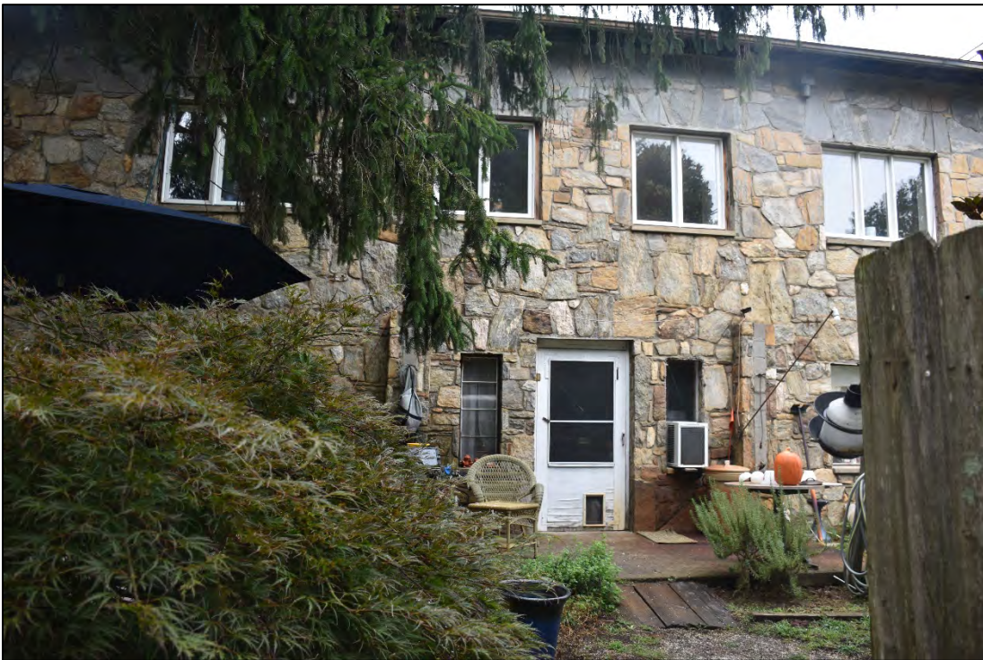
Figure 2.29. Meadow's Store and Apartments (BN6343), facing north.
