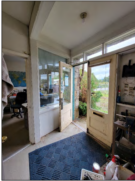
Figure 2.13. Meadow's Store and Apartments (BN6343), store interior, facing northwest.
