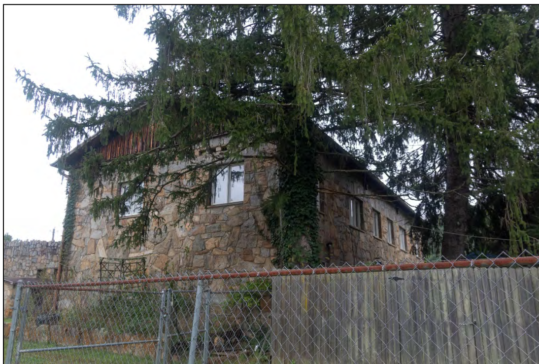
Figure 2.27. Meadow's Store and Apartments (BN6343), facing northeast.
