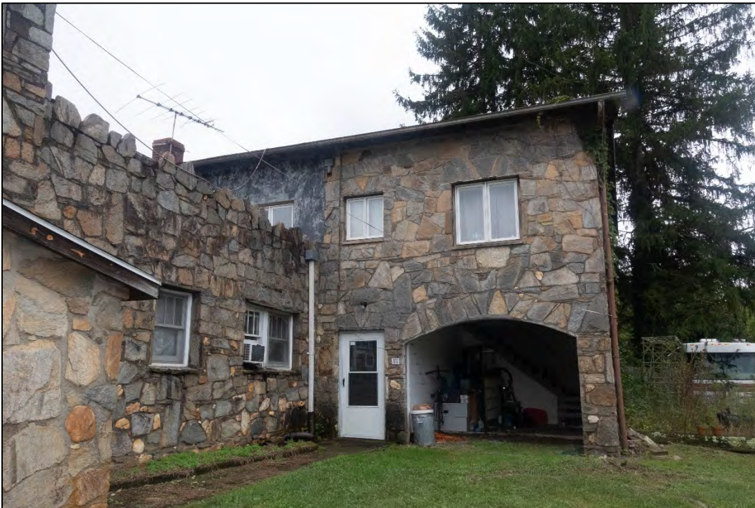
Figure 2.20. Meadow's Store and Apartments (BN6343), facing southeast.
