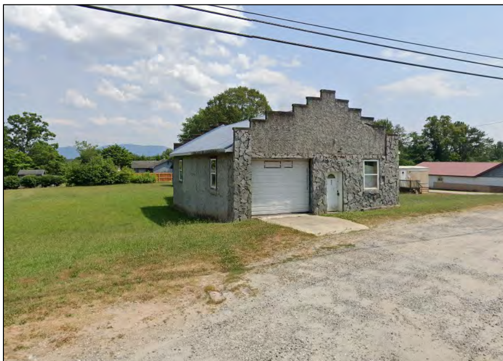
Figure 2.53. Commercial Building (BK0374), facing south (image from Google Streetview).
