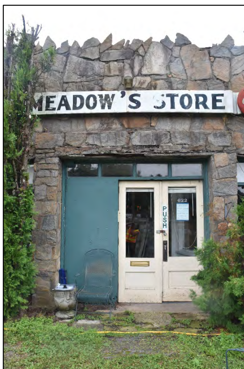
Figure 2.4. Meadow's Store and Apartments (BN6343), entry detail, facing south.
