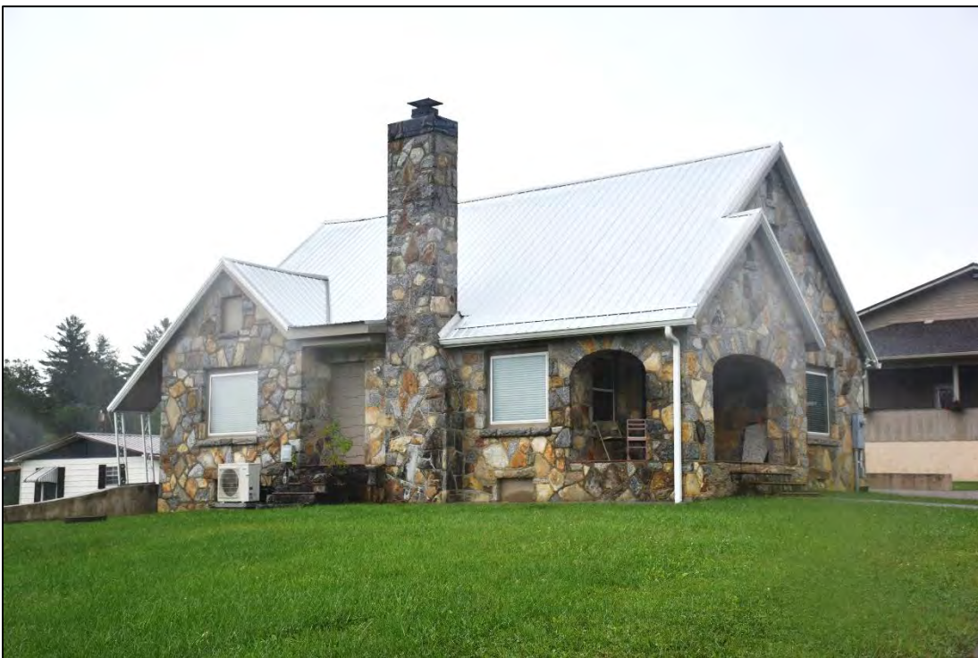
Figure 2.50. Unsurveyed House at 384 Fruitland Road, facing northeast.
