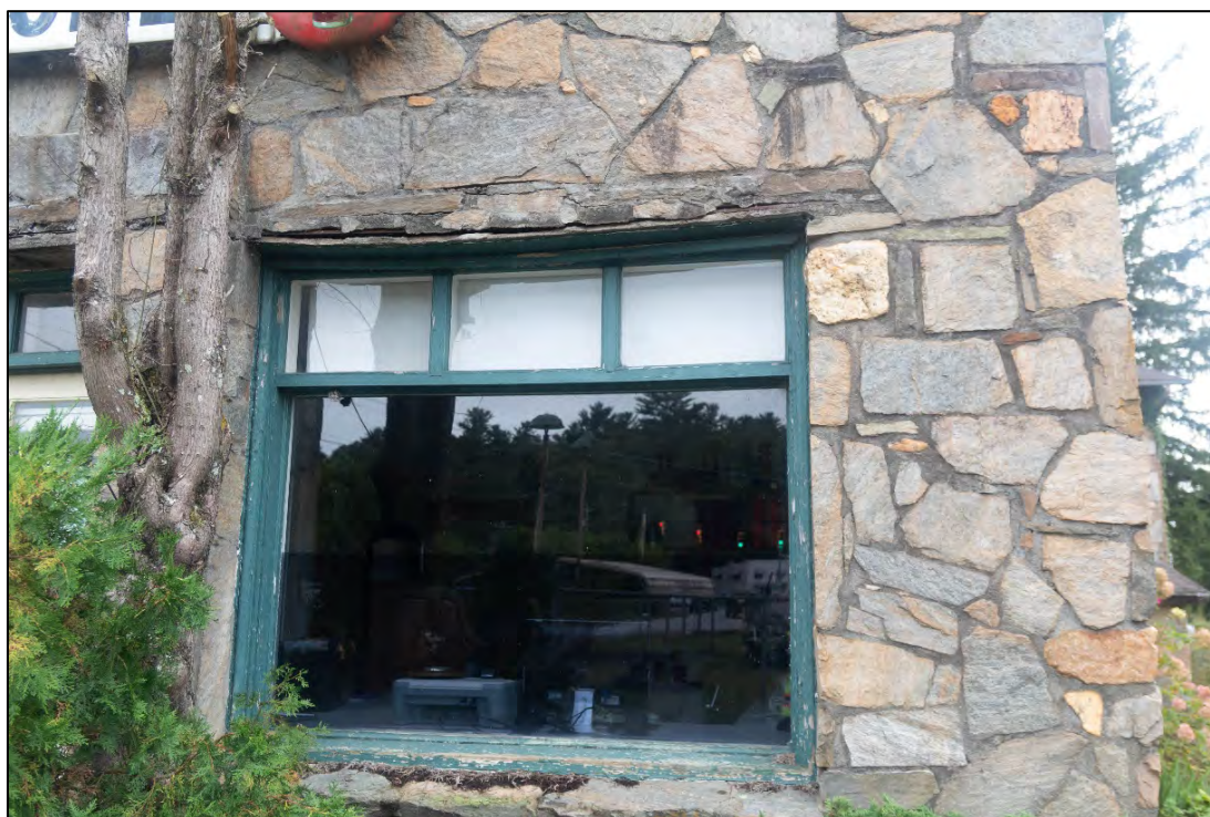
Figure 2.5. Meadow's Store and Apartments (BN6343), store window detail, facing south.
