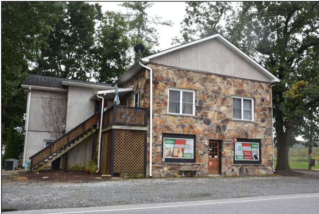
Figure 2.57. Unsurveyed Structure, 1206 Dana Road, Hendersonville, facing southwest.
