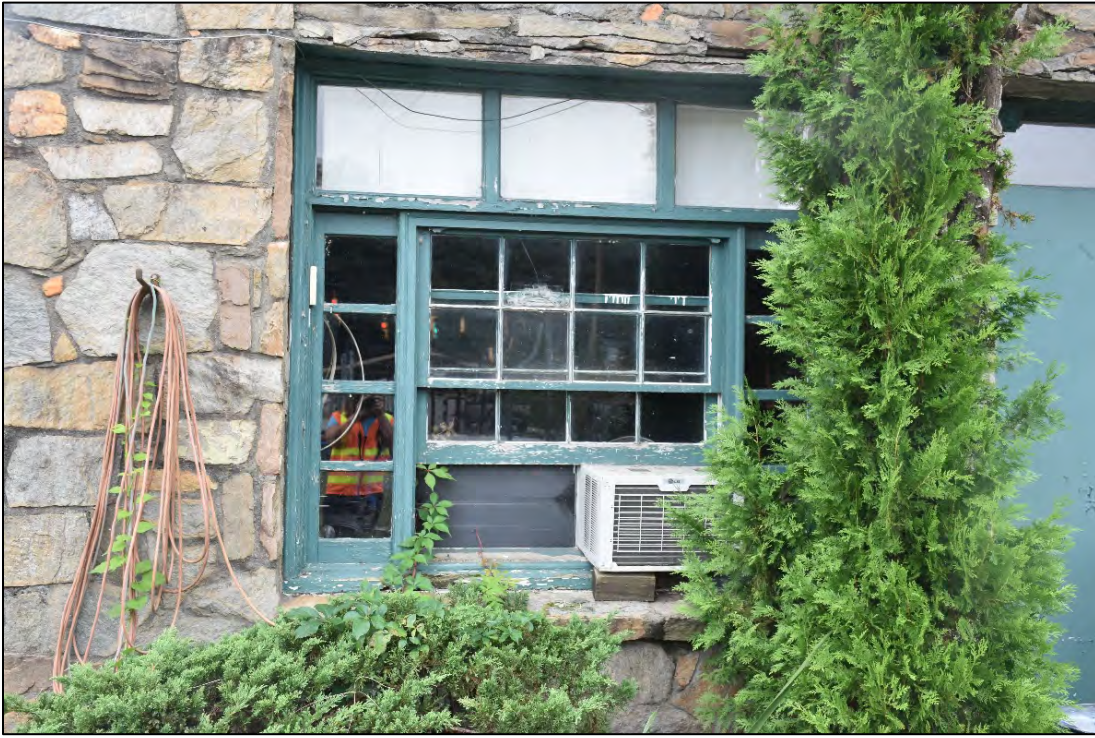
Figure 2.6. Meadow's Store and Apartments (BN6343), store window detail, facing south.
