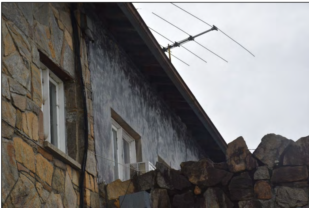
Figure 2.19. Meadow's Store and Apartments (BN6343), wall detail, facing southwest.
