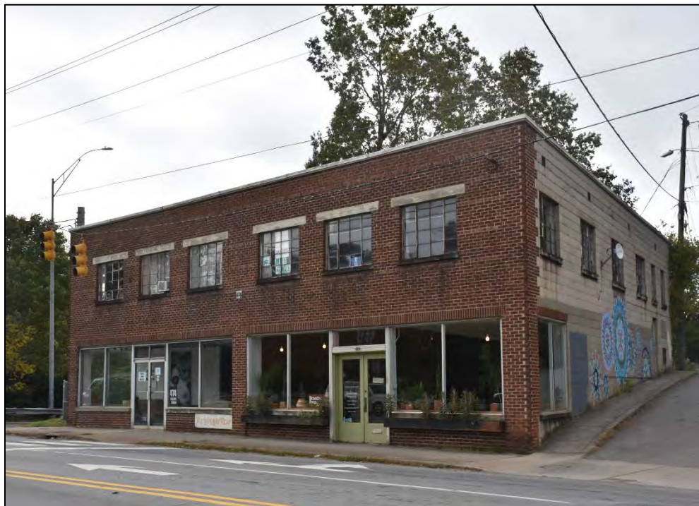
Figure 2.38. Meadow's Dry Goods Shop (BN4931), Asheville, facing southeast.
