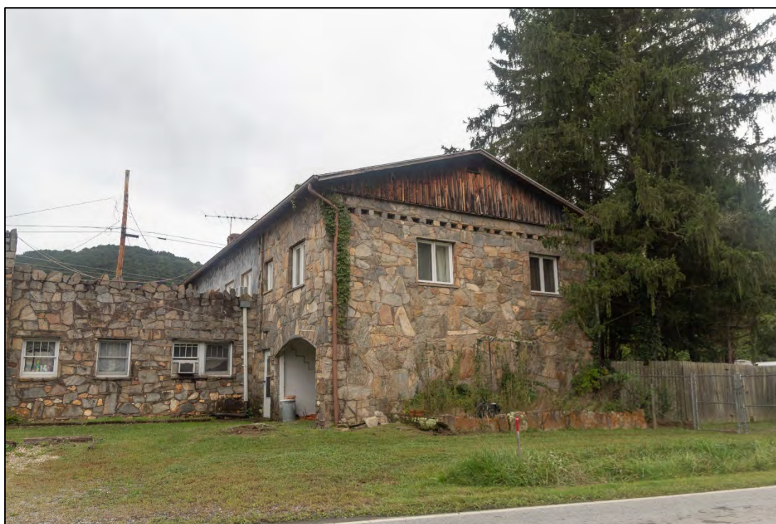
Figure 2.23. Meadow's Store and Apartments (BN6343), facing southeast.
