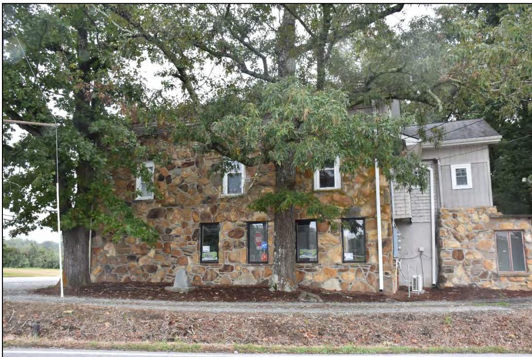
Figure 2.58. Unsurveyed Structure, 1206 Dana Road, Hendersonville, facing east.
