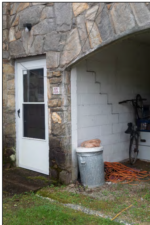
Figure 2.21. Meadow's Store and Apartments (BN6343), apartment door and garage, facing southeast.
