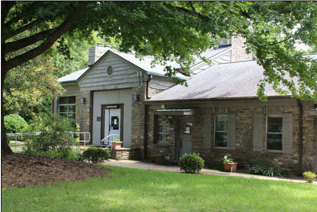
Figure 2.47. Lutheridge (BN6304), Efrid Hall, facing southeast
