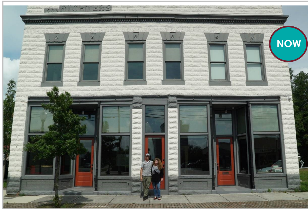
Richter Building Wilmington, New Hanover County
