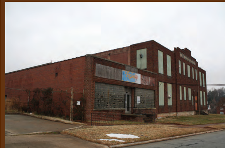
Mock, Judson, Voehringer Company Hosiery Mill now eligible for historic mill tax credits
