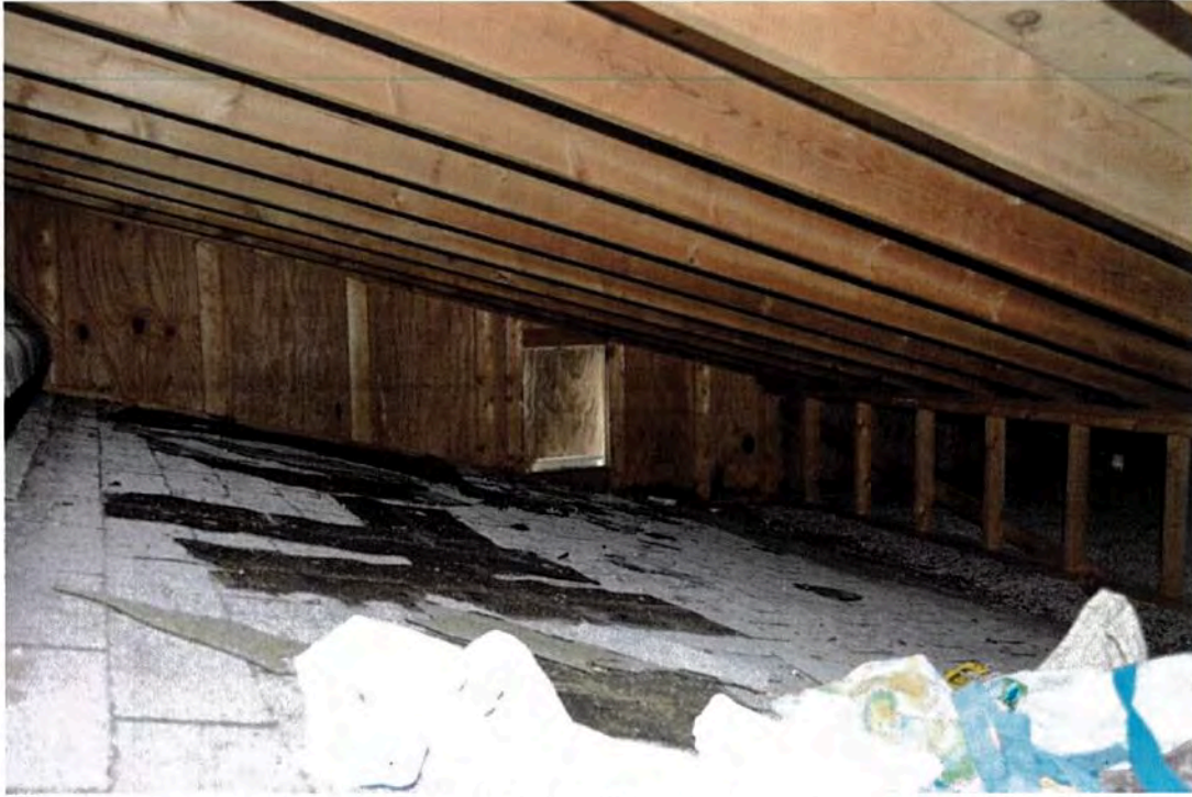
Fig. 7. 1970 rear addition attic showing first period shed roof. View looking west
