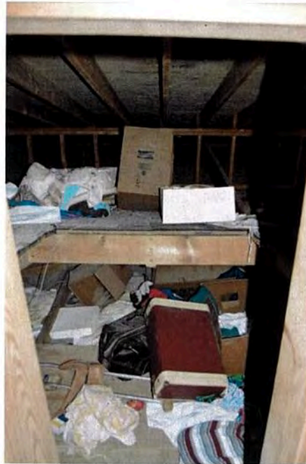
Fig. 20. 2 nd floor bathroom – view looking east from landing
