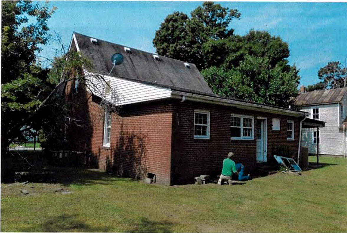
Fig. 6. View looking northeast from rear showing 1970 ten-foot addition.
