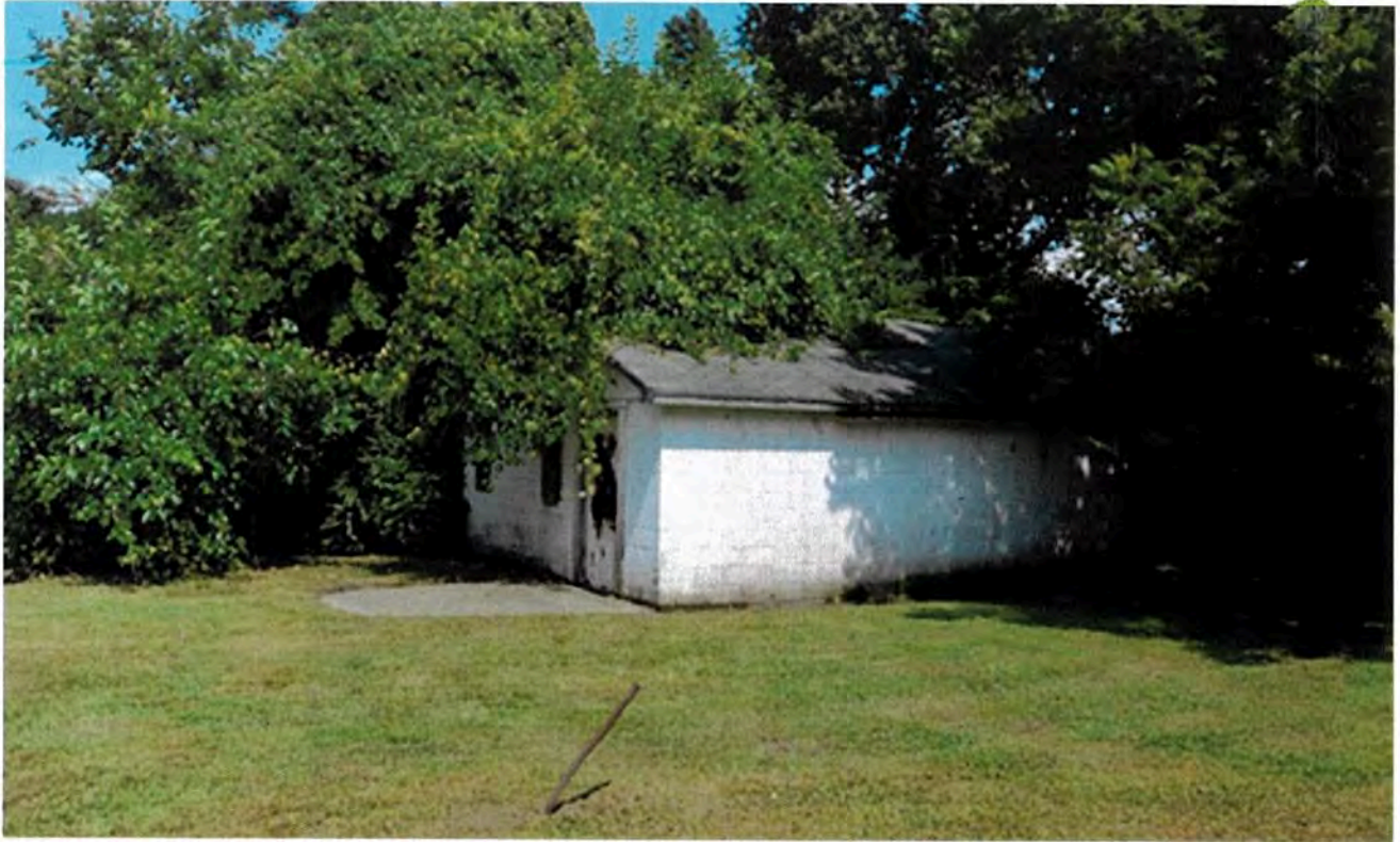
Fig. 24. Concrete-block outbuilding – northwest corner of property
