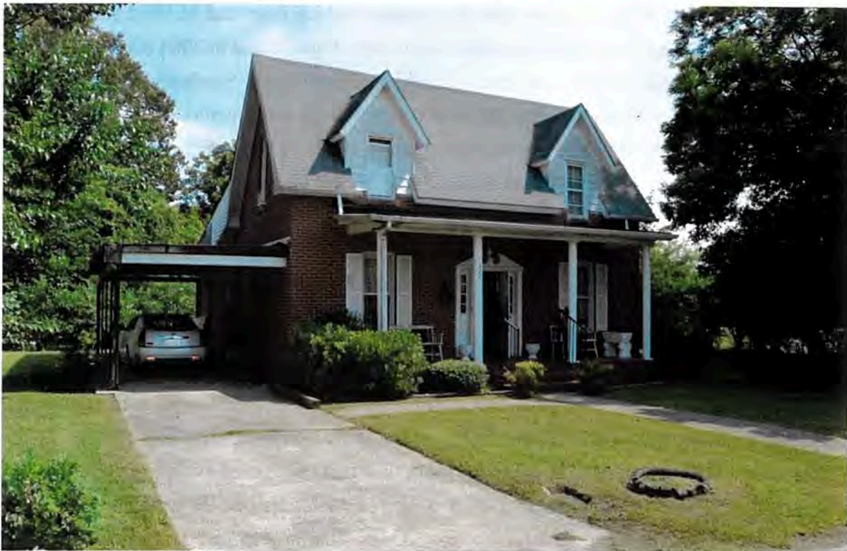
Fig. 2. South elevation – Brick veneer, carport, porch, shutters, and front entry dates from the 1970 renovation.
