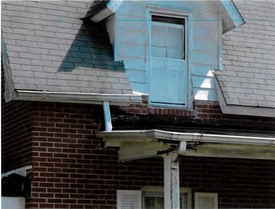
Fig. 23. Southwest corner of front porch.
