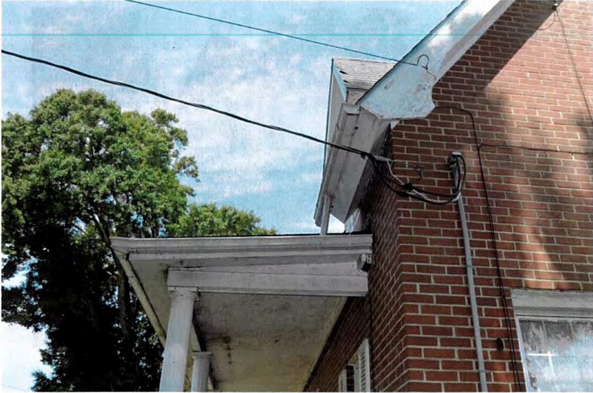
Fig. 3. Porch and cornice detail – east side
