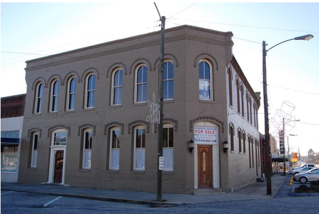
Corner of East H and South Thirteenth streets, looking south
