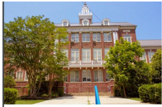
MAIN BUILDING at Durham School of The Arts
